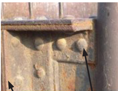
Plaque contre-joint rivet
